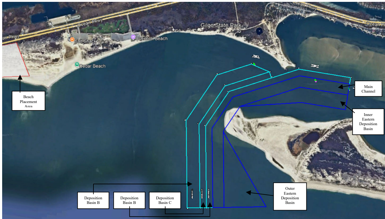
Figure 1: Fire Island Inlet; approximate location of area to be dredged
